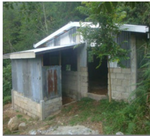
On-going construction of the Animal House at CSAC Experiment Farm
