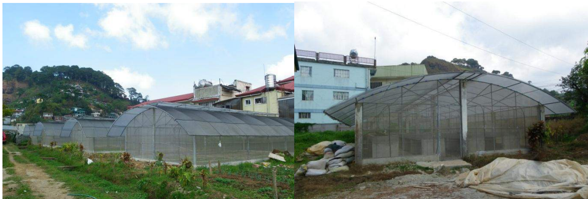
Five units of greenhouses at the Floriculture Project were installed for the conduct of research on ornamentals as well as to serve as laboratory for students of the College of Agriculture
