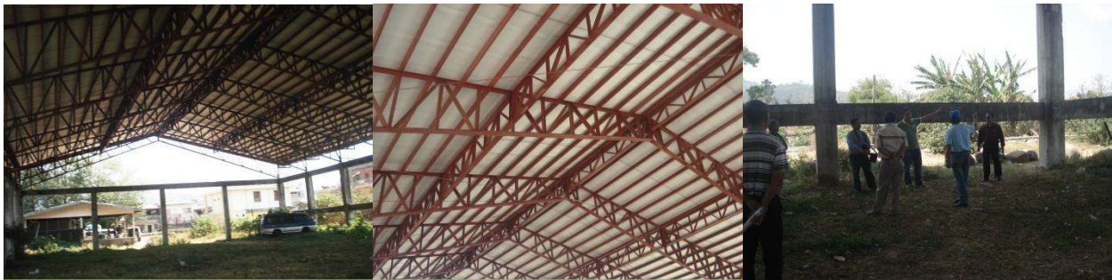
The Buguias Campus Multipurpose Hall was enclosed
