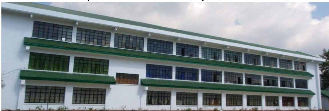
The College of Veterinary Medicine Building was repaired and repainted to facilitate learning and teaching
