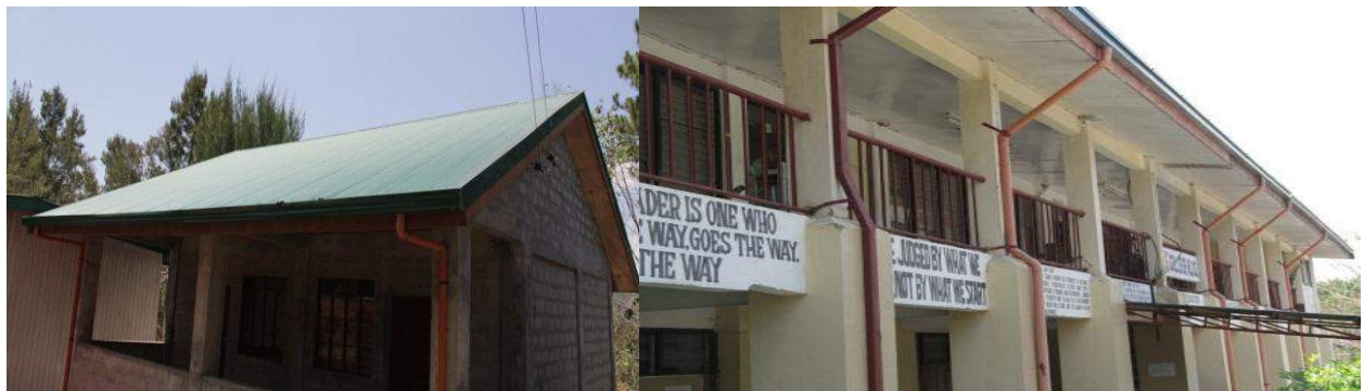
The dilapidated gutters of 6 buildings of the campus were replaced
