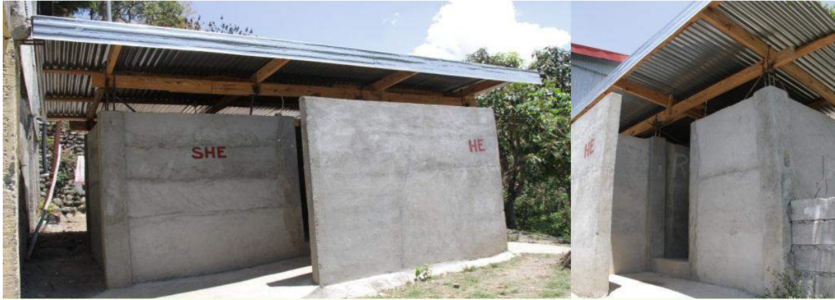
Two latrines for the Science and Health Office were constructed
