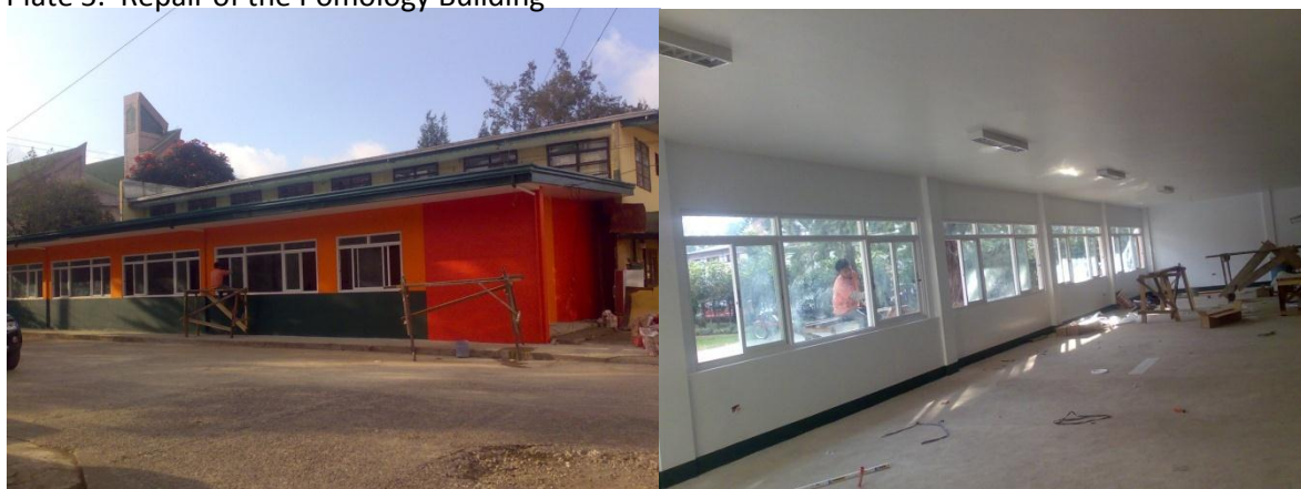
Plate 5. Repair of the Pomology Building
