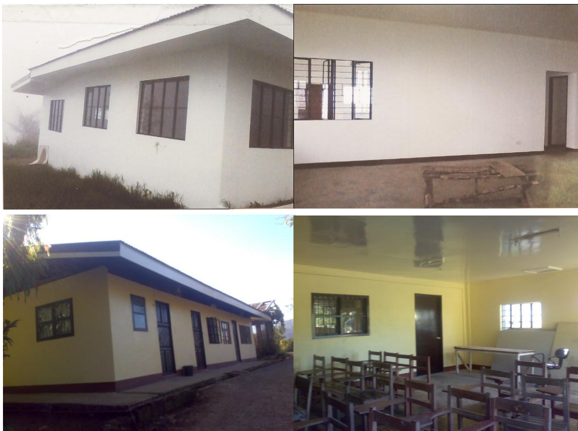
Plate 4. Repair of the Institute of Highland Farming Systems and Agroforestry
